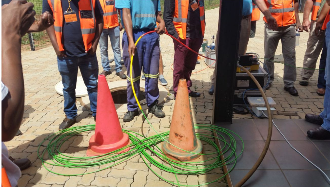
Center blowing (mid-span blowing) Figure-eighting the cable
